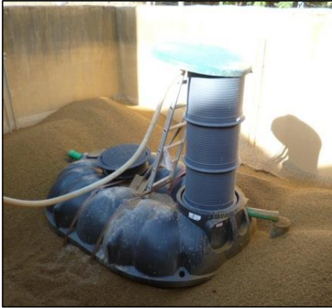
During backfilling and water filling with inlet/outlet fittings shafts
