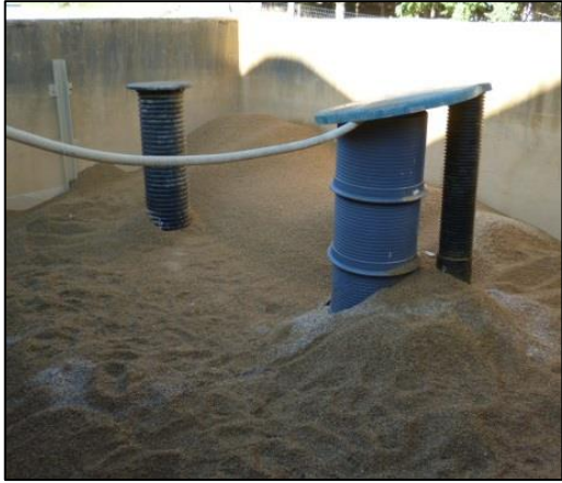
During backfilling and water filling with inlet/outlet fittings shafts
